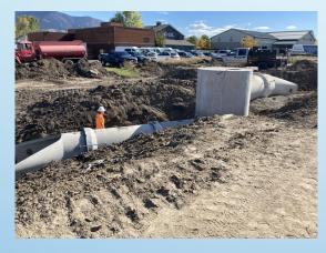
"The City of Bozeman's storm sewer serves two purposes: (1) mitigate flood risk by collecting runoff from streets, parking lots, alleyways, and other hard surfaces, and (2) treat stormwater by capturing sediment, trash, and other pollutants in their sumps. The storm sewer requires regular maintenance, including vacuuming and flushing, to stay functional."
