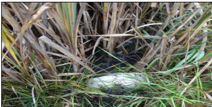
Image 4 - Obstructed inlet pipe
