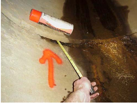
Figure 2.3: Marking pipe joint separation
