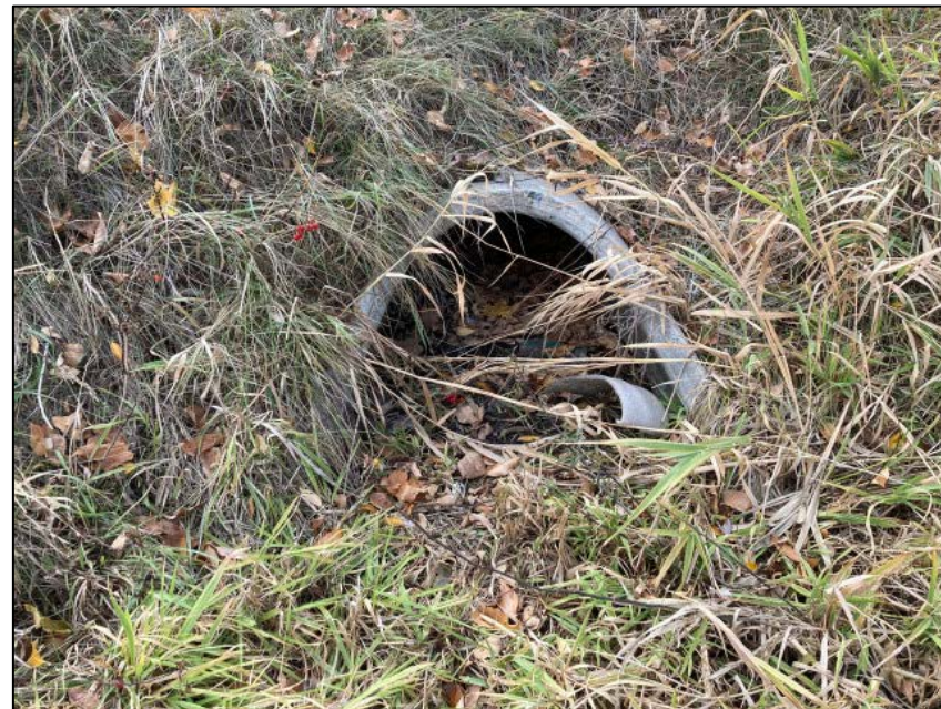
Image 2 Detention Facility Inlet showing sediment accumulation
