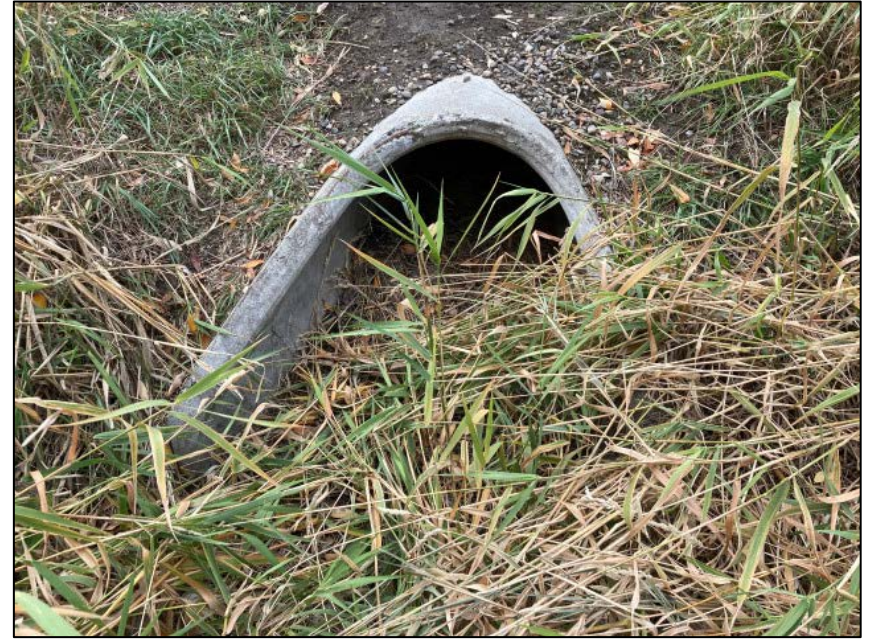
Image 4 Detention Facility Outfall with vegetation and sediment accumulation
