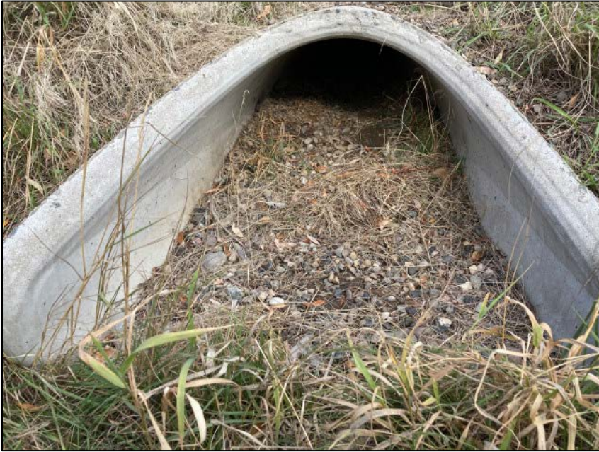
Image 3 Detention Facility Outlet showing sediment accumulation
