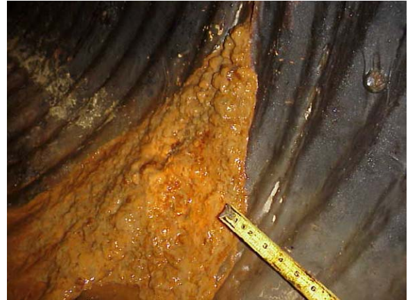
Figure M3.2: Soil entering open pipe joint.
