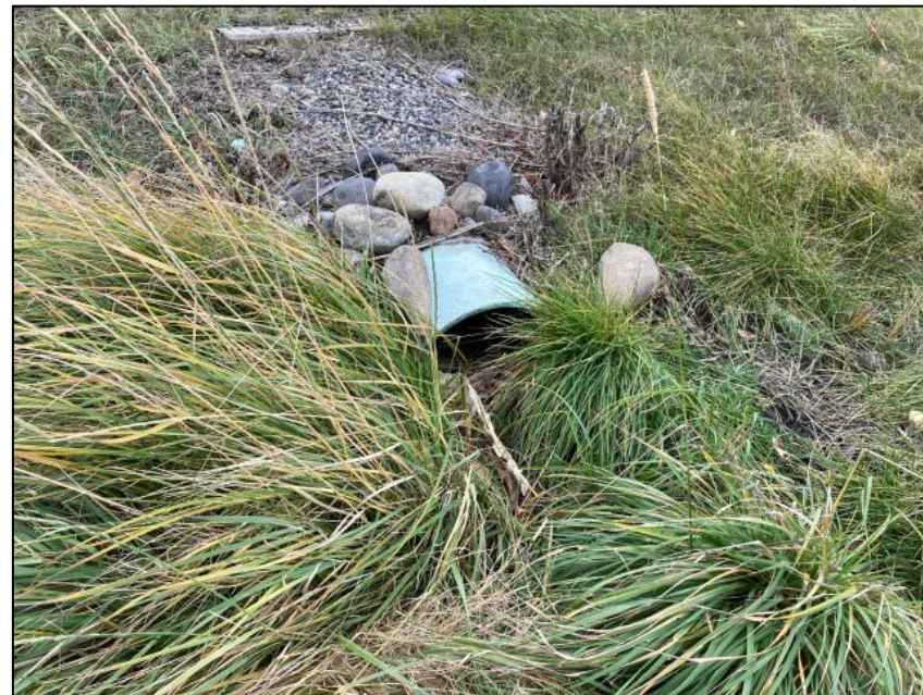
Image 2 Overgrown grass at facility inlet
