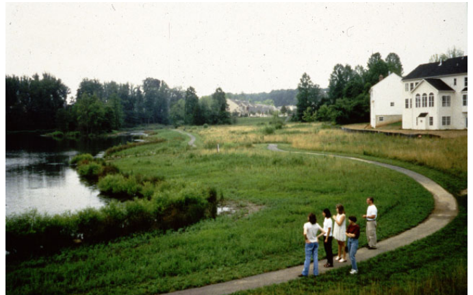
Figure M4.4: Vegetated buffer.
