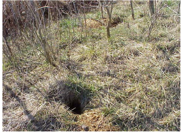
Figure 1.17: Animal burrow in pond embankment.
