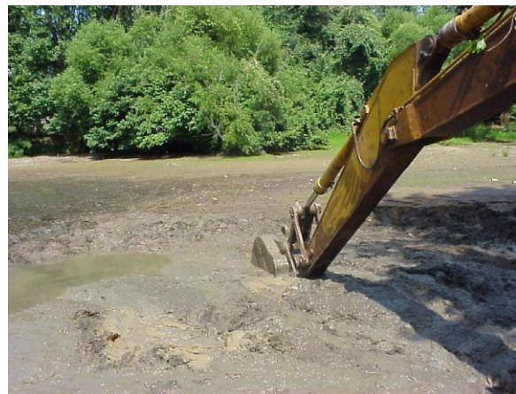
Figure M5.4: Mechanical dredging with backhoe.
