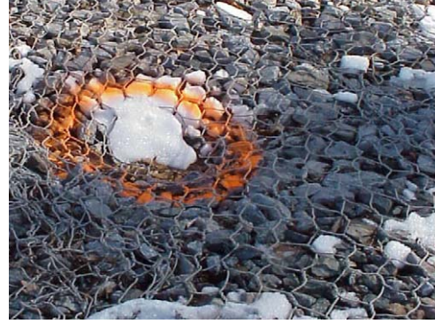
Figure 2.4: Marking a hole in gabion fabric
