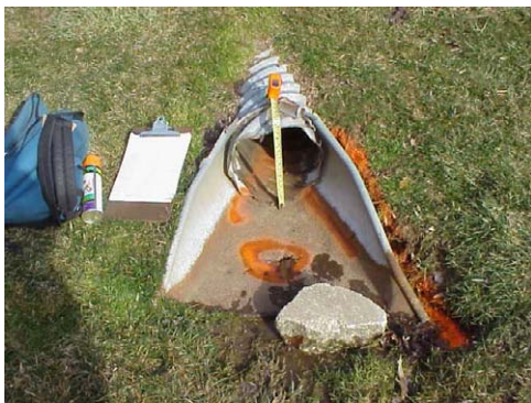
Figure 2.1: Marking outfall deficiencies.
