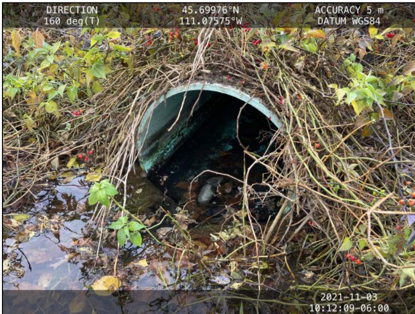
Image 3 Southern detention facility inlet, water flowing into basin from around and outside of pipe
