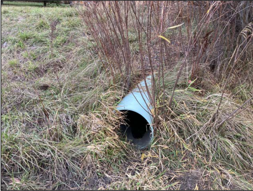
Image 3 Outlet pipe within detention facility showing willow growth encroachment
