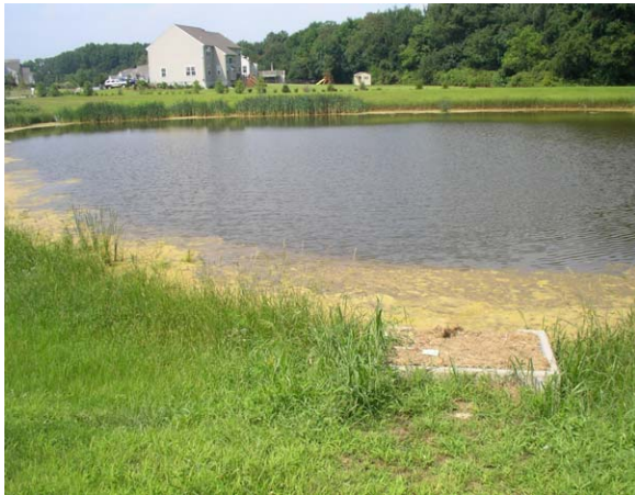
Figure 1.2: Flattop riser covered with debris.
