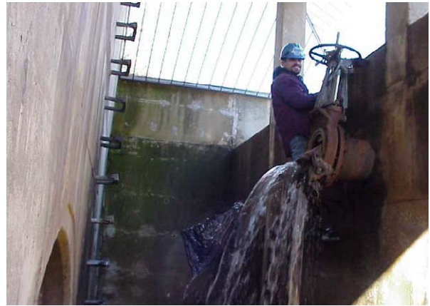
Figure M2.1: Clogged valve.
