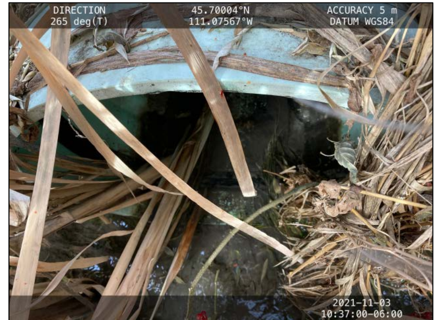
Image 4 Detention facility outlet; flowing water
