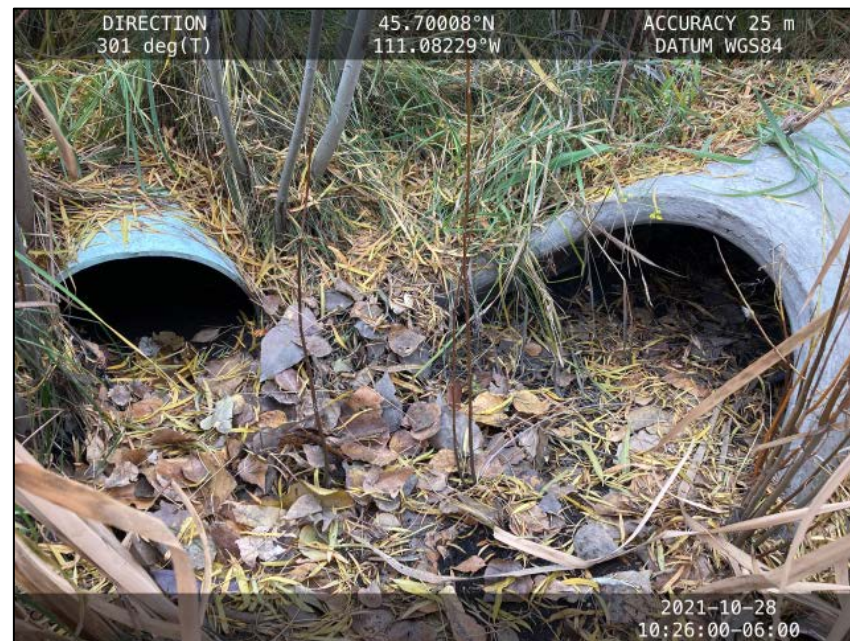
Image 2 Inlets at west end of detention facility, partially clogged with sediment
