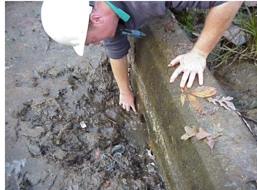
Figure M2.3: After clog is removed.
