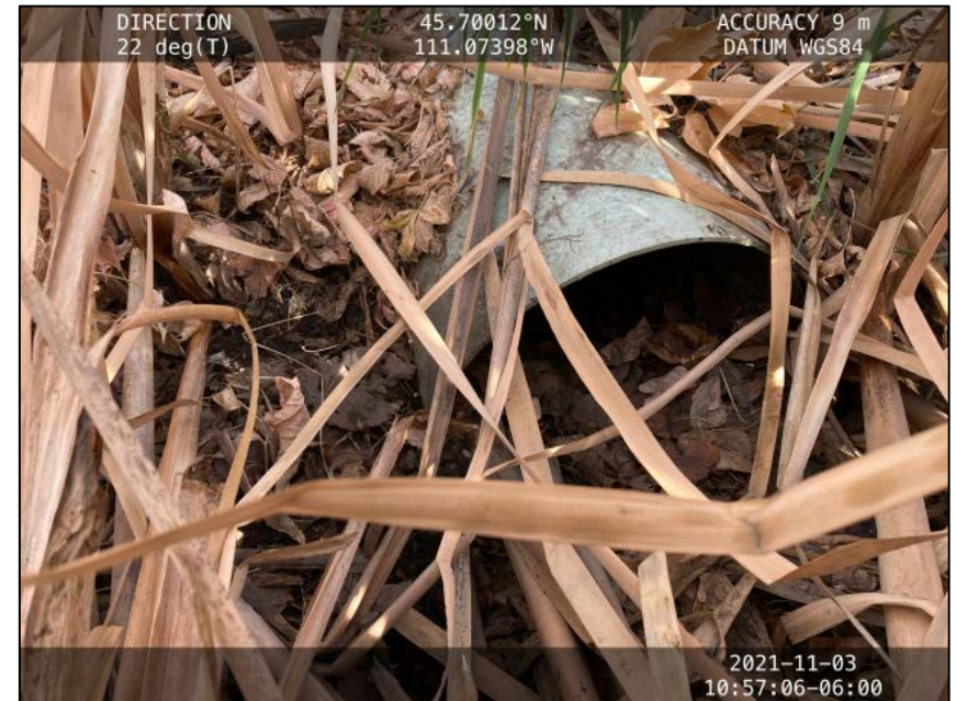
Image 2 Retention Facility inlet from Baxter Ln; more than ½ filled with sediment
