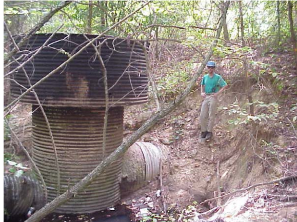
Figure 1.5: Severe erosion around riser and barrel
