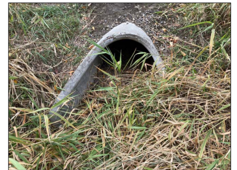
Image 4 Detention Facility Outfall with vegetation and sediment accumulation
