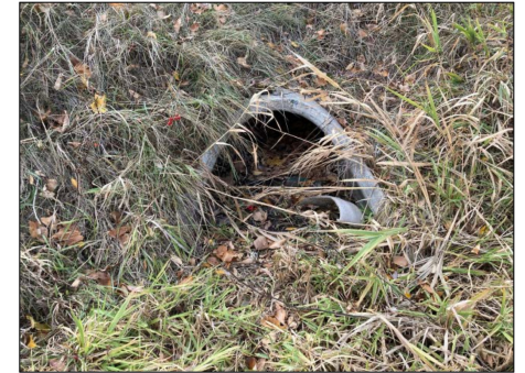
Image 2 Detention Facility Inlet showing sediment accumulation
