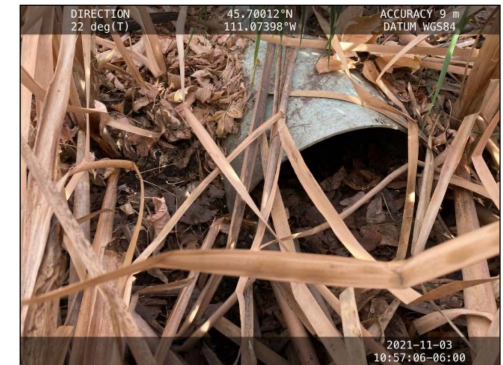
Image 2 Retention Facility inlet from Baxter Ln; more than 1/2 filled with sediment
