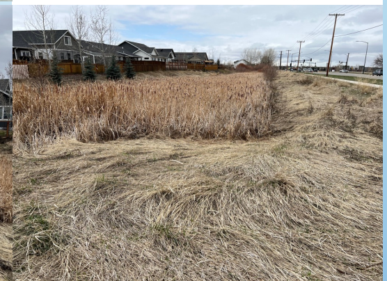
Image 3 Detention Facility outlet; inhibited flow and vegetation growth.
