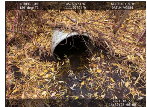
Image 2 Detention Facility Inlet from Tschache Rd to 'forebay'
