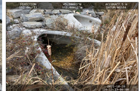
Image 3 Detention Facility outlet; inhibited flow and vegetation growth.
