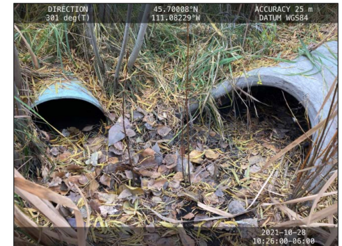
Image 2 Inlets at west end of detention facility, partially clogged with sediment
