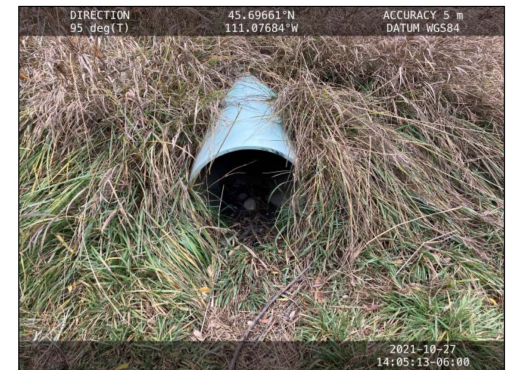
Image 4 Detention Facility Outfall
