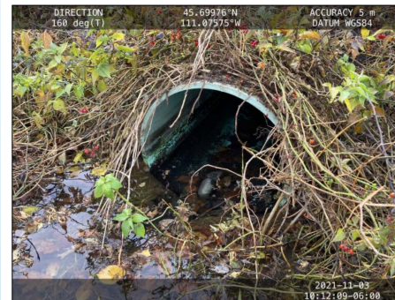
Image 3 Southern detention facility inlet, water flowing into basin from around and outside of pipe
