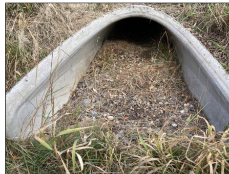
Image 3 Detention Facility Outlet showing sediment accumulation
